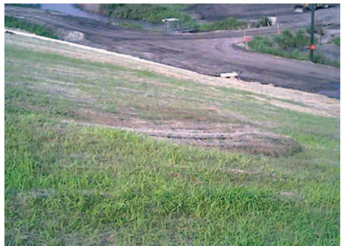
**Photo 2.** Surface slump on a section of the cover without the drainage composite installed. The drainage composite was placed on either side of the slump, but not beneath.
