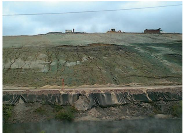
**Photo 1.** Slumps and erosion rill on a 2H:1V slope of a paper mill sludge landfill.
