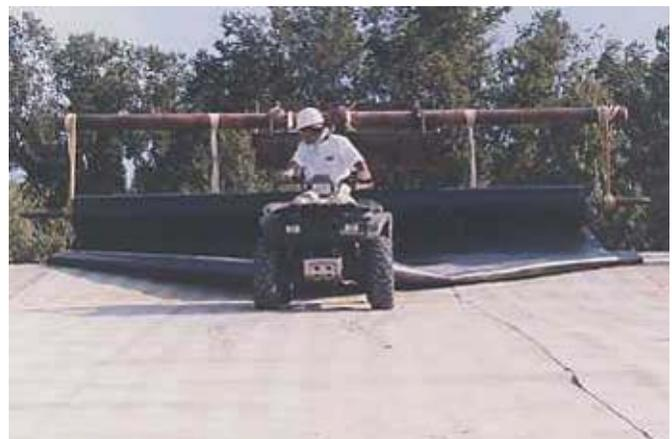
**Photo 2:** Deployment of a geomembrane over a GCL with an all-terrain vehicle.
