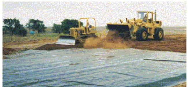
*Photo 4: Soil cover placement over a GCL.*
