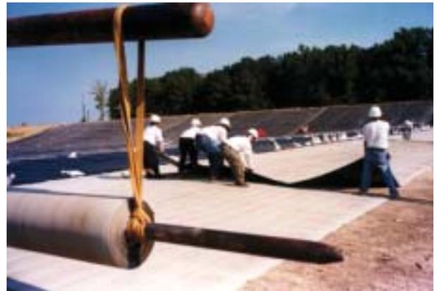
**Photo 3:** Final manual alignment of a deployed GCL.
