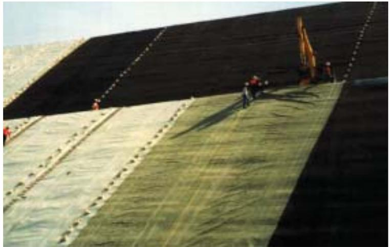
**Photo 1:** Installations of a GCL over a protective geotextile cushion.
