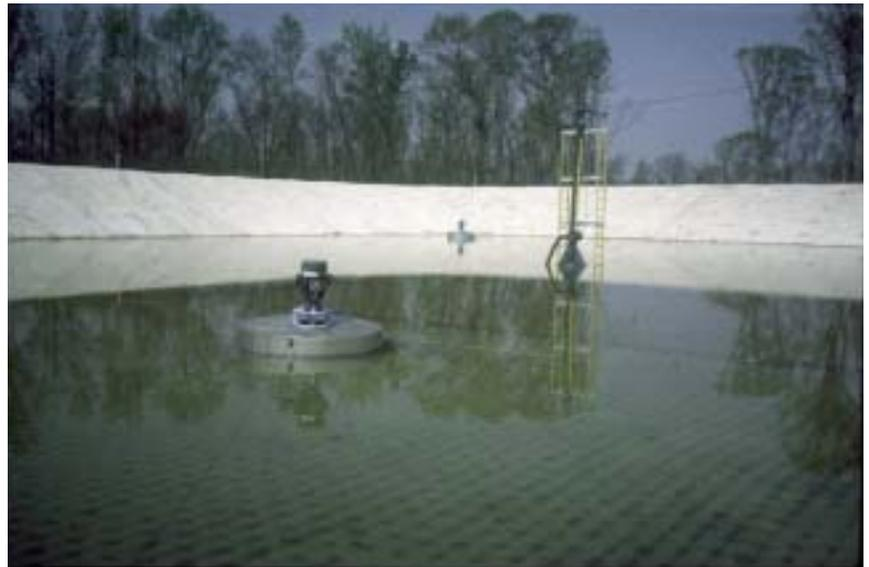
**Photo 2.** Fabri-form protected liner in an environmental pond.
