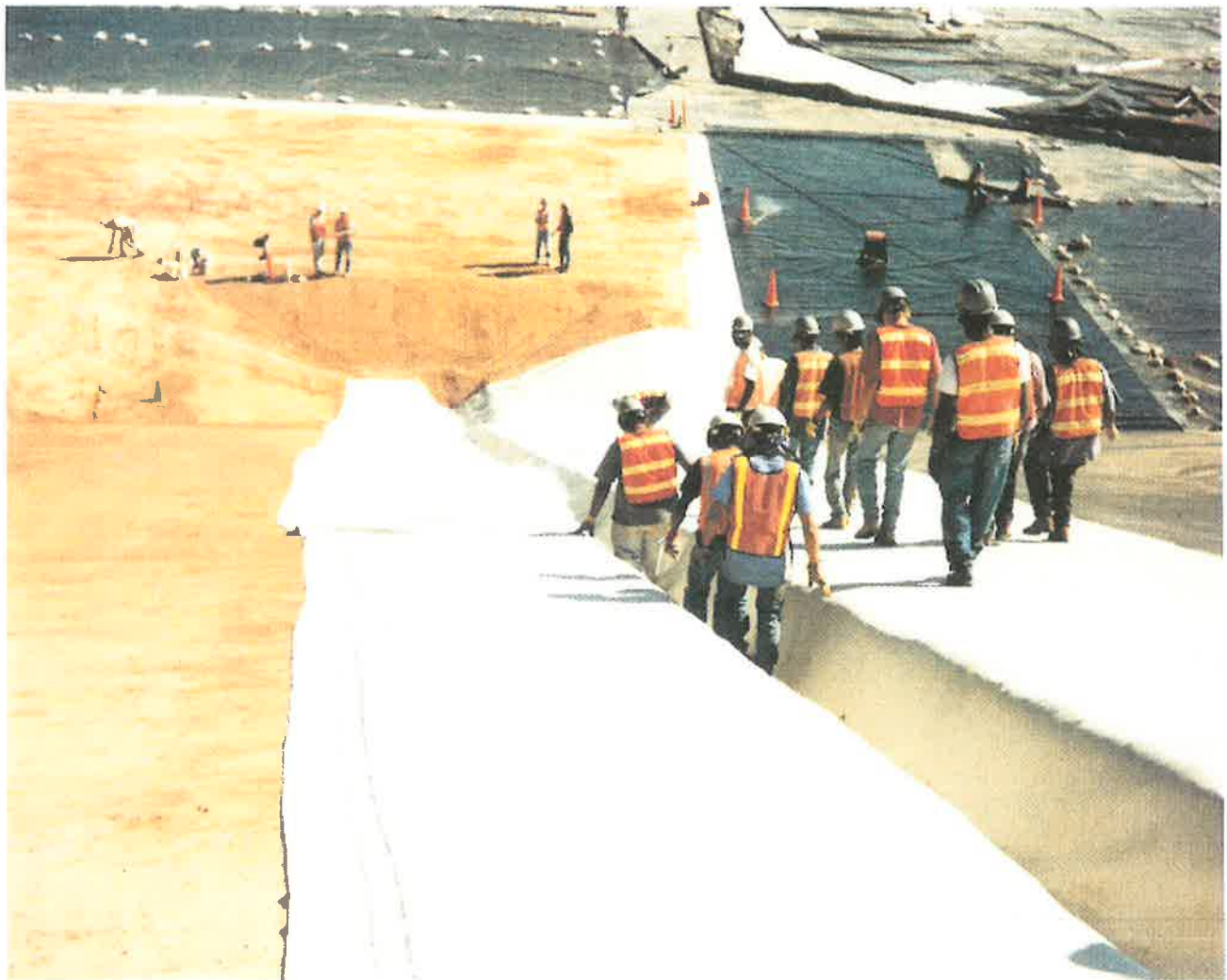
Placing GCL in the west upslope trench of the Monticello repository.
