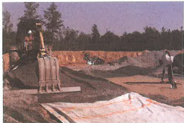
Photo 2. A modified screed was used to remove aggregate without damaging underlying samples.
