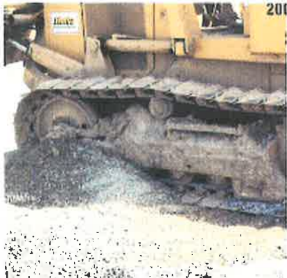
Photo 3. A D7 dozer makes a typical stone-placement maneuver.
