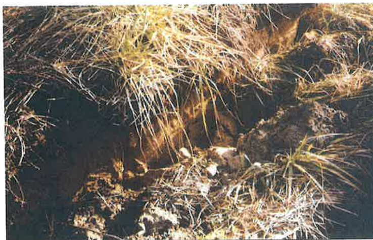
Photo 2. Crack observed in cover.
