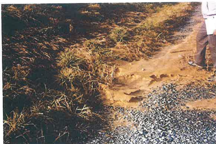
Photo 1. Silt drainage at toe of slope.
