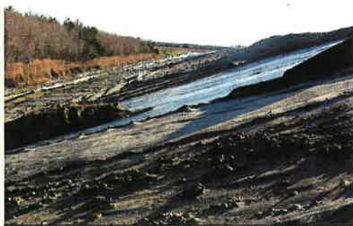
Photo 1. Initial slope failure.
